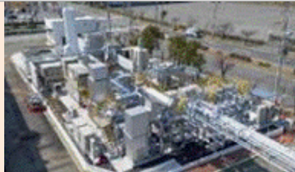
Hydrogen power generation facility (hydrogen CGS) constructed on Port Island in Kobe City
