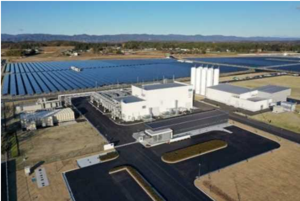
Alkaline electrolyser plant in Fukushima
