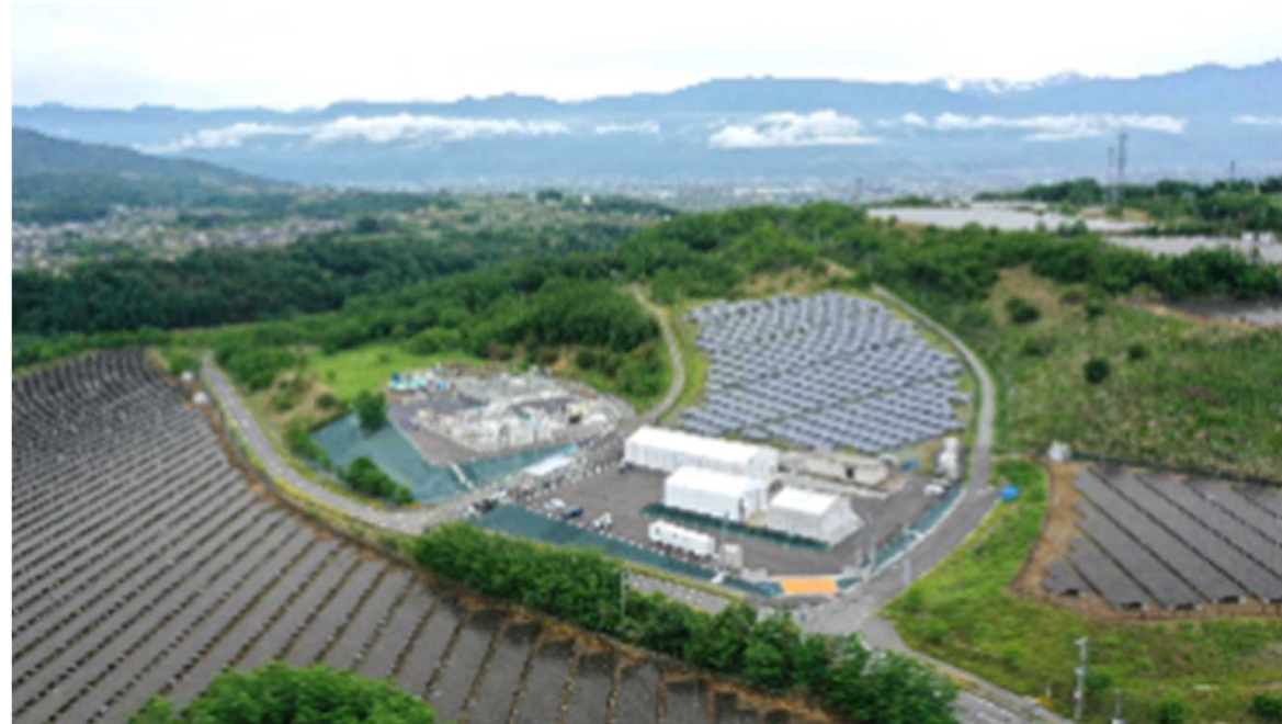
PEM electrolyser plant in Yamanashi
