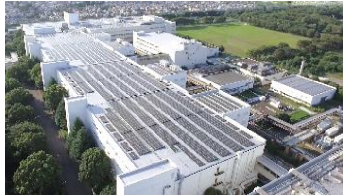
Solar panels installed at the Abiko Plant
