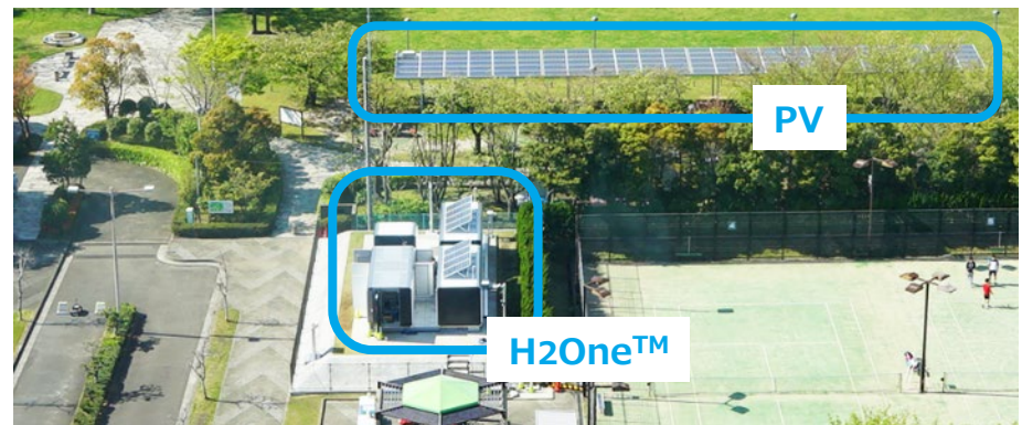
Footprint: approx. tennis court 1 field including PV
