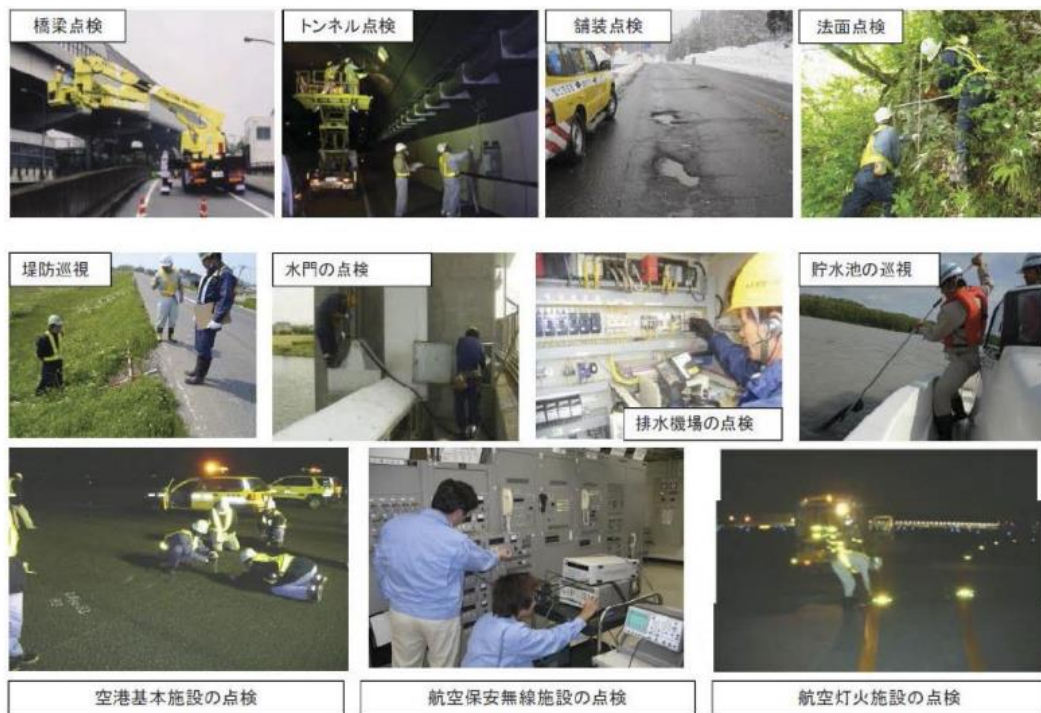
Figure 4-38 Various forms of visual inspections carried out in Japan (MLIT, 2016)
