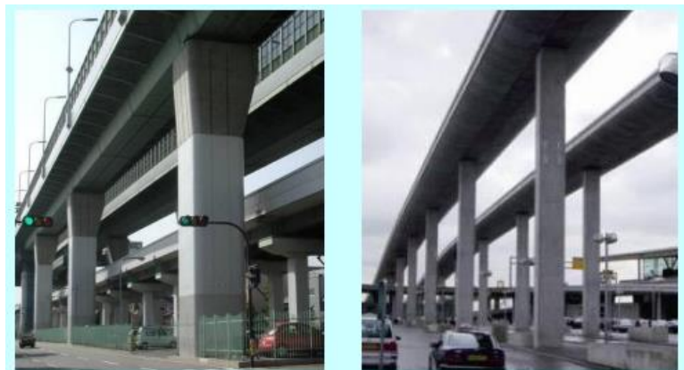
Figure 4-36 Struttred supports in Japan (left) and France (right) (MLIT, 2015)
