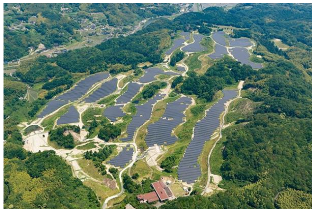
Solar panel in Yamaguchi Pref., Image from TOKYO Gas website
