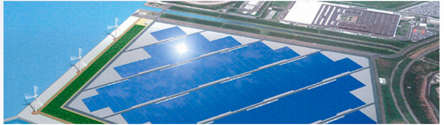
Tahara (Aichi Pref.) Megasolar PV plant
